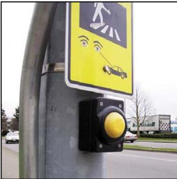
The flashing yellow lights are activated by a pedestrian pushing a button at the curb. These flashing lights are timed to stay on long enough to allow pedestrians to cross the street.
